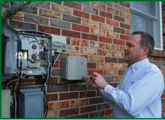
BVU Network Service Specialist Chris George checks a FTTH connection at a residence.
