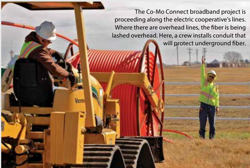
The Co-Mo Connect broadband project is proceeding along the electric cooperative's lines. Where there are overhead lines, the fiber is being lashed overhead. Here, a crew installs conduit that will protect underground fiber.
