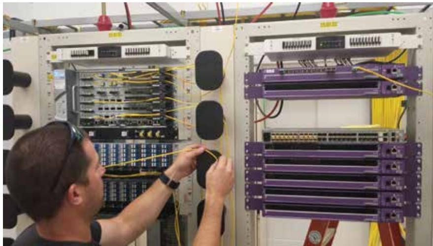
An HBC technician feeds fiber lines to Calix E7 OLTs in the main network operating center.
