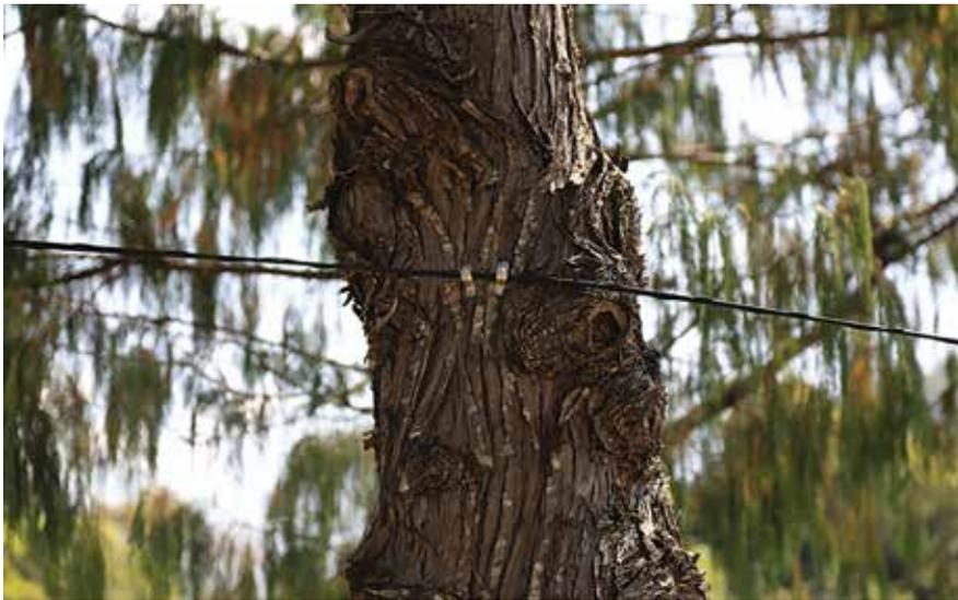
An aerial installation of L.1700 fiber in Bhutan makes use of a conveniently located tree.
