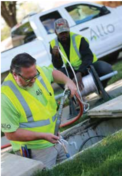
Allo's fiber will reach every premises in Lincoln..
