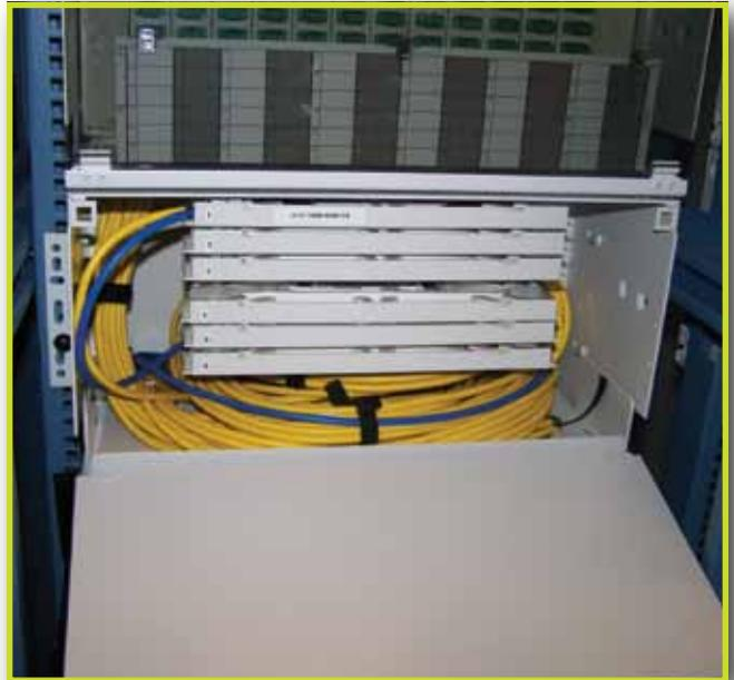
Under-desk deployment: Pigtail cable is routed down a wall.
