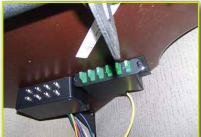
Front faceplate with bulkhead adapters is oriented toward the user, allowing for patching to equipment on the desk.
