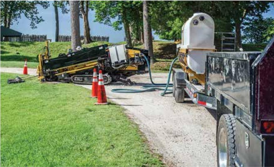
Since 2019, Cox has installed 13,000 linear feet of directional boring, pedestals, ground vaults and fiber runs on Jamestown Island.
