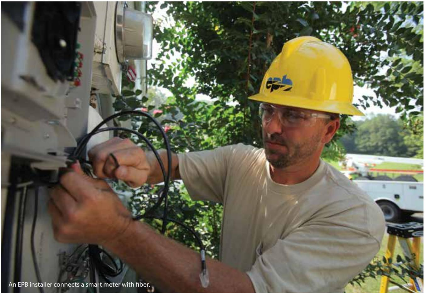
An EPB installer connects a smart meter with fiber.
