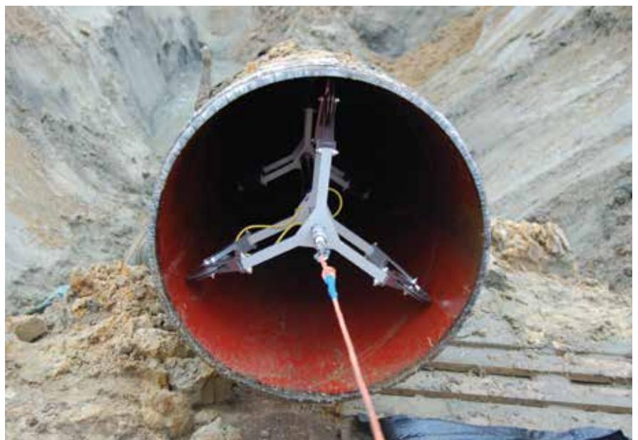
The Condux duct-mapping solution at work
