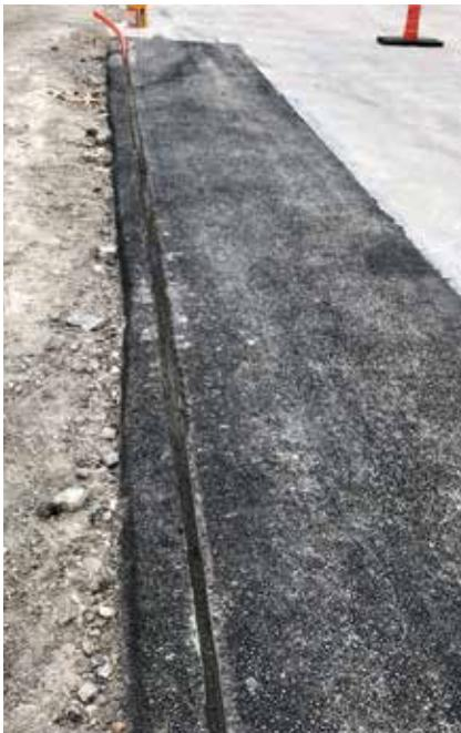
A demonstration of “reinstatement,” the refilling of microtrenches after the conduit has been placed in it. Corbel Communications, which hosted the conference at its Austin, Texas facilities, is one of three suppliers, along with Crafcro and GCP Applied Technologies, that has invented specialized material for reinstatement.
