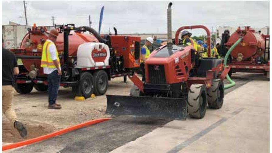
The highlight of the conference was a series of live demonstrations of microtrenching techniques, including the sawing of a trench, the placement of conduit, and the use of various materials for reinstatement.
