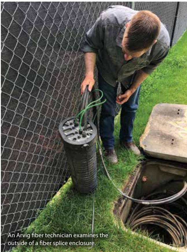
An Arvig fiber technician examines the outside of a fiber splice enclosure.
