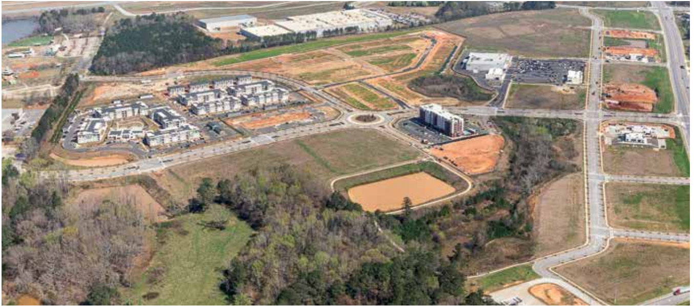
AT&T Fiber will deliver high-speed broadband to all residents and businesses in Covington Town Center.
