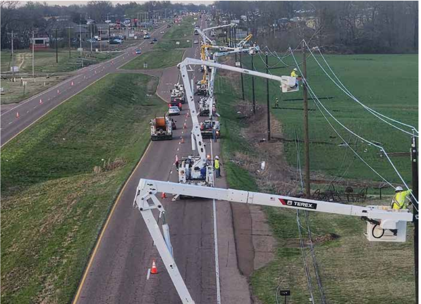
STEMC and Aeneas are jointly building and expanding a fiber network to bring broadband communications to the region.
