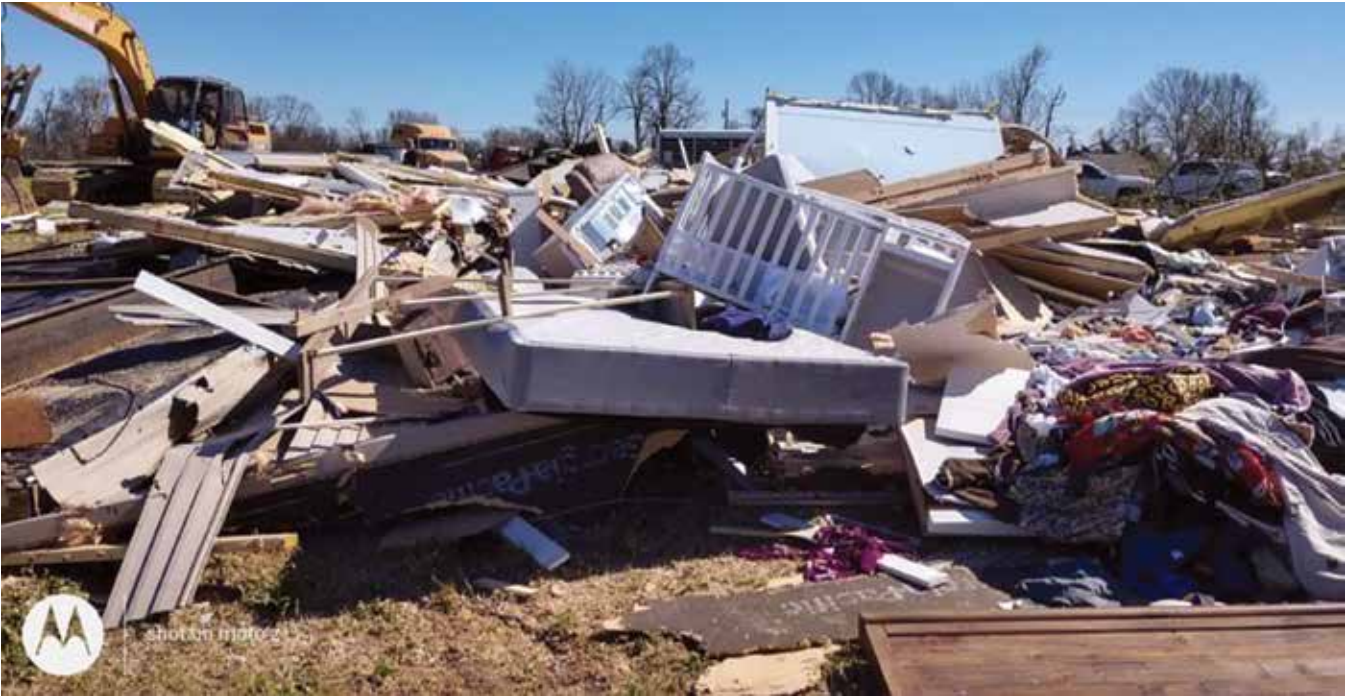
STEMC's partnership with Render and Irby Utilities helped the electric cooperative recover from an F3 tornado quickly.
