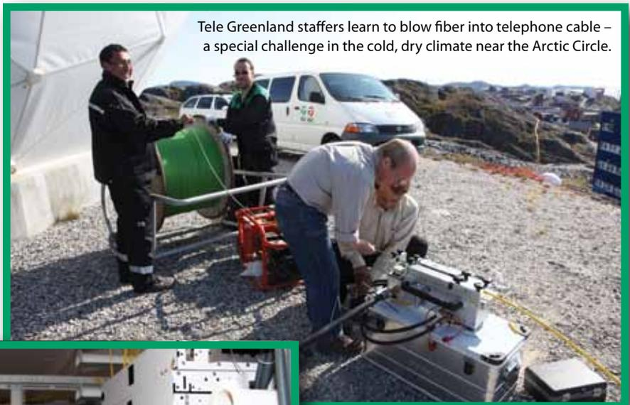
Tele Greenland staffers learn to blow fiber into telephone cable – a special challenge in the cold, dry climate near the Arctic Circle.
