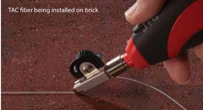
TAC fiber being installed on brick
