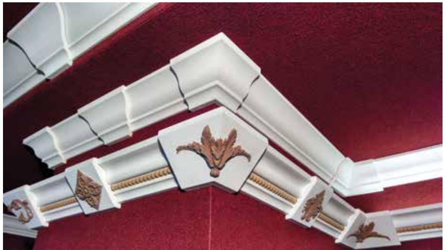
Seam covers and mitered corner blocks are snapped on over the faceplate.
