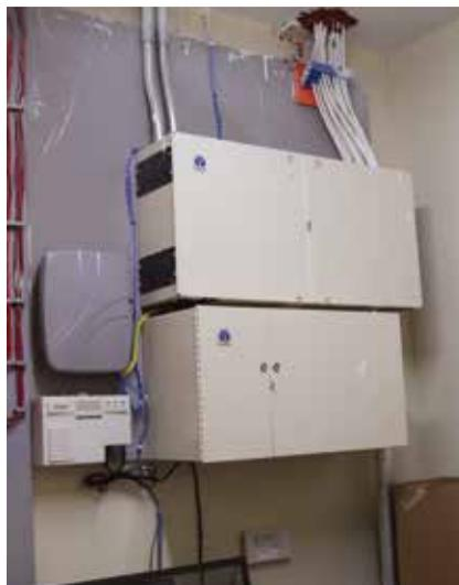
Clearfield FieldSmart fiber entrance cabinet (top) loaded with fiber splice trays and FieldSmart Wallbox with 1x32 splitters (bottom)
