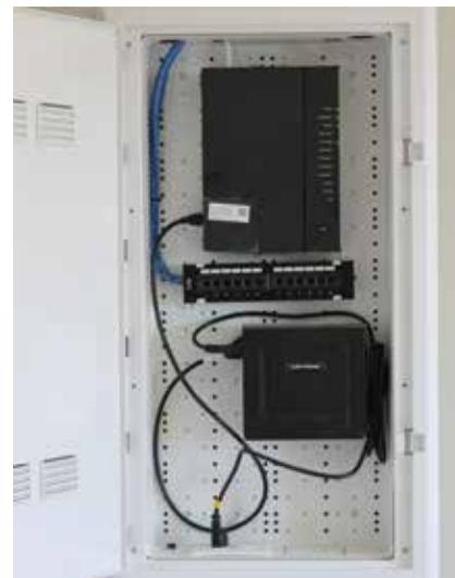
Fiber-fed structured wire deployment (Calix ONT on top, Ethernet distribution patch panel below it and power supply at the bottom)
