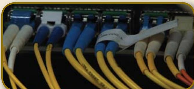
Fiber jumpers connecting to the core data routers.
