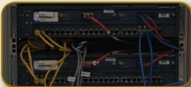
Data switch showing redundant multimode uplinks.
