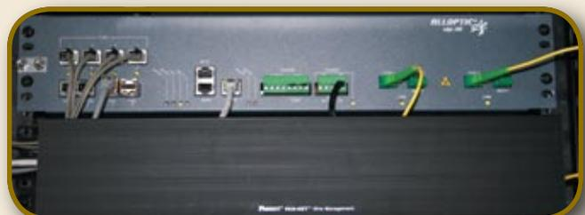
The Alloptic ONT housed inside the power cabinet provides 25 Mbps Internet connectivity and telephone service to each yacht.
