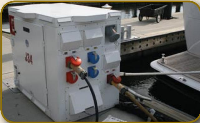
The power pedestal on the dock supplies 480v, 240v and 208v electrical service to each boat. The big cables are the electrical supply; the smaller blue cable is the Cat 5 line providing Internet connectivity to the boat.
