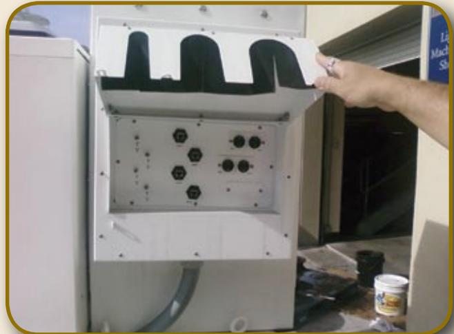
The customer sees this interface at the slip for data, phone and television jacks, if needed. Gaskets protect the cabinet from the weather. The ONT inside this cabinet gives off enough heat to evaporate any moisture.
