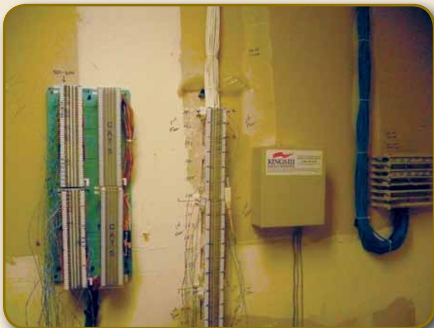
A termination block and switching panel is located in each closet.
