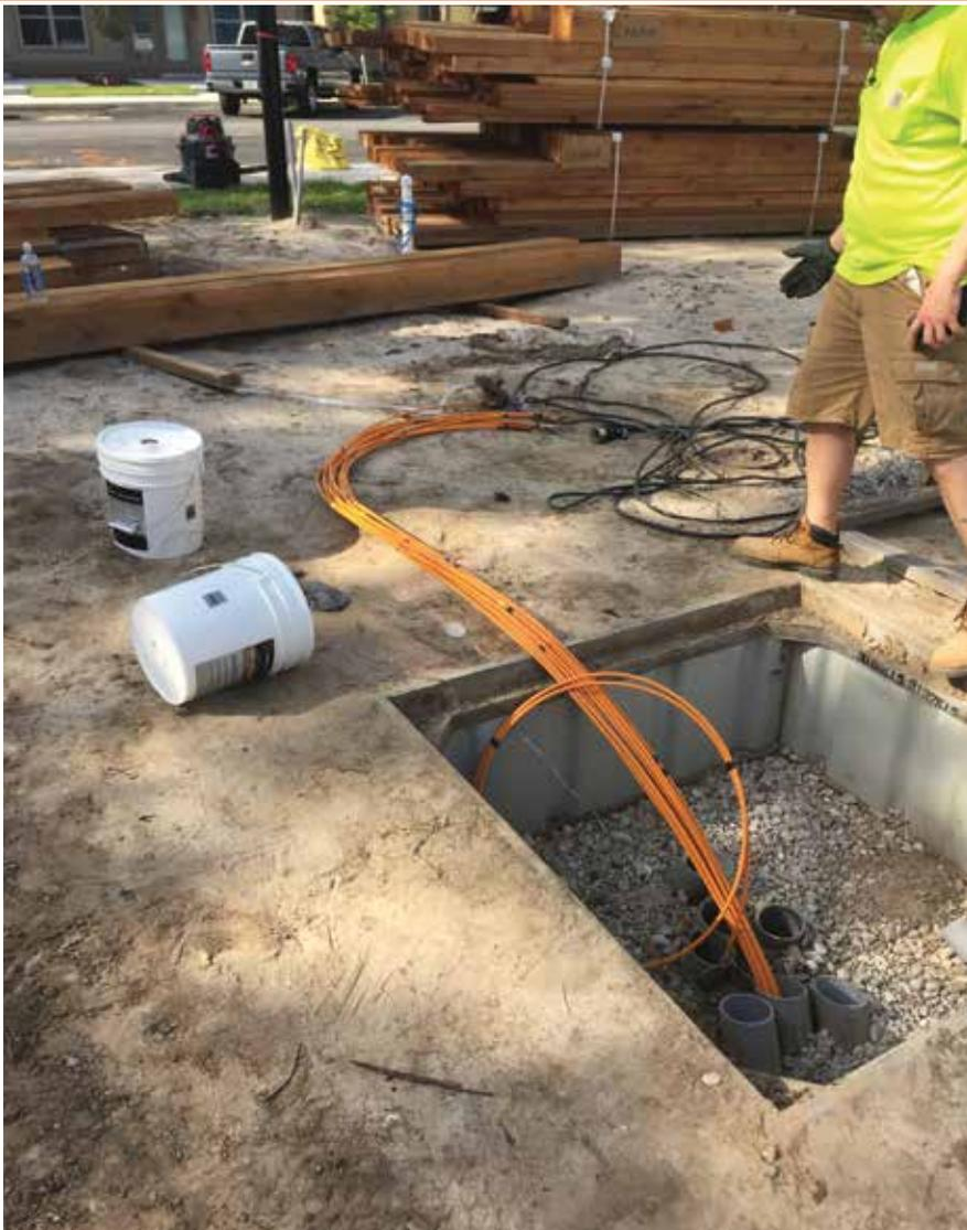
A technician buries TuffDuct microduct for a Miniflex fiber installation at a college housing complex in Florida.
