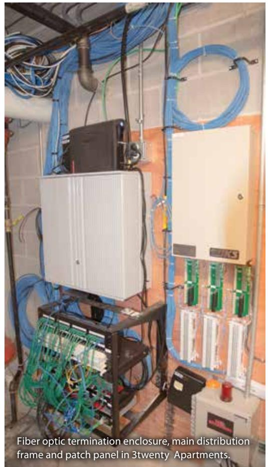
Fiber optic termination enclosure, main distribution frame and patch panel in 3twenty Apartments.
