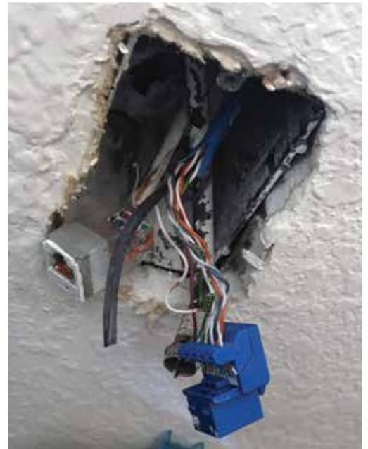
Figure 1: A student apartment wall jack after several years of painting and repairs
