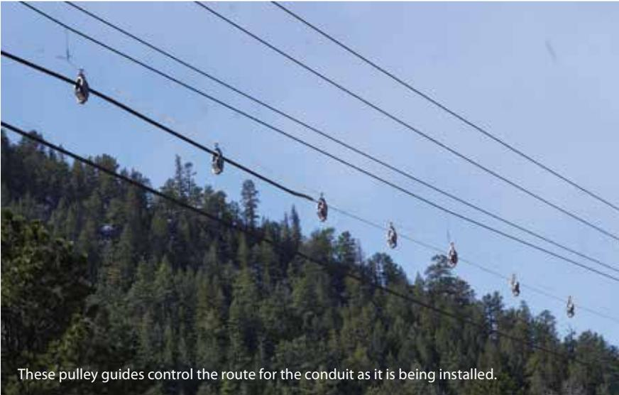
These pulley guides control the route for the conduit as it is being installed.
