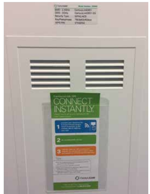
A nonmetallic media panel reduces interference with Wi-Fi.
