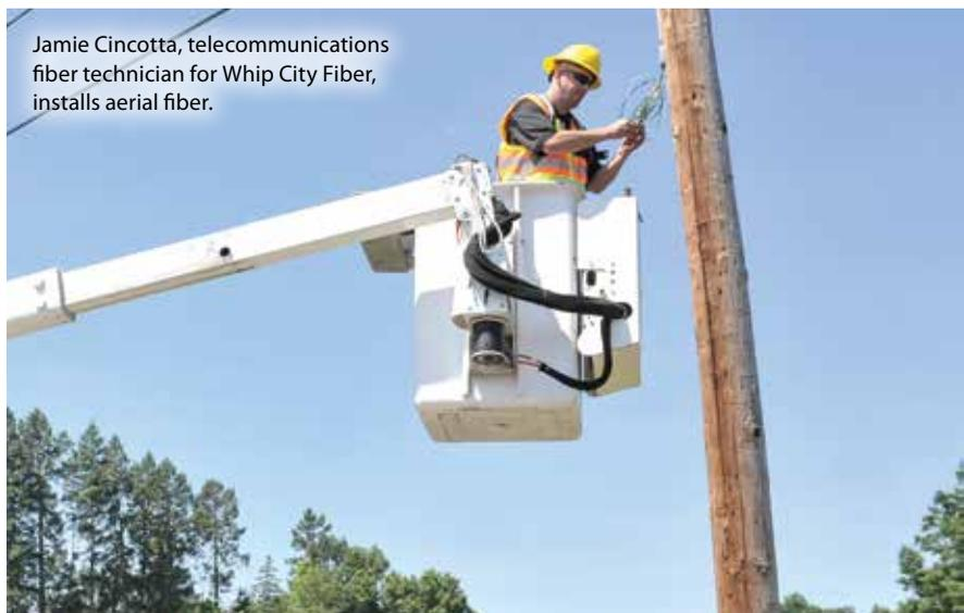
Jamie Cincotta, telecommunications fiber technician for Whip City Fiber, installs aerial fiber.
