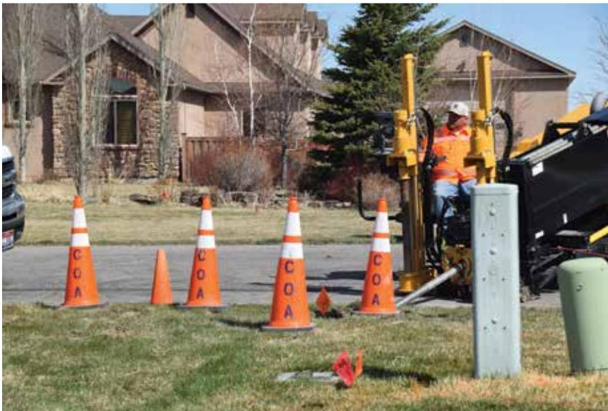
Installing fiber duct and underground vaults in a right-of-way in a residential neighborhood
