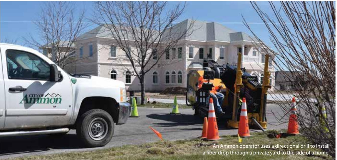
An Ammon operator uses a directional drill to install a fiber drop through a private yard to the side of a home.
