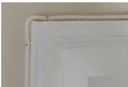
Figure 7: Inside the customer premises, fiber may be stapled to the wall, mounted on the wall surface or track-mounted.
