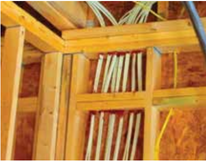
Figure 4: Conduits installed for fiber distribution
