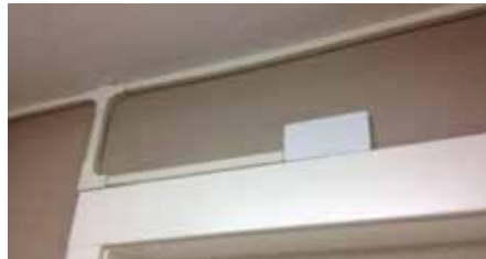
Figure 5: In an existing building, cable can be installed above a drop ceiling, beneath molding, on a wall surface or on the building exterior.
